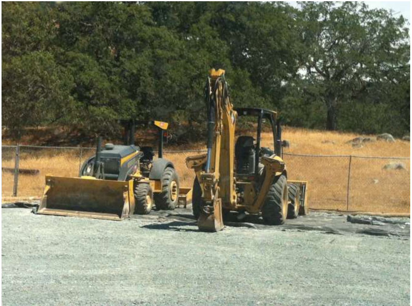
Photo 6: Visqueen was staged under equipment at the Santa Ysabel Yard in order to prevent any potential equipment leaks from contaminating soils.
