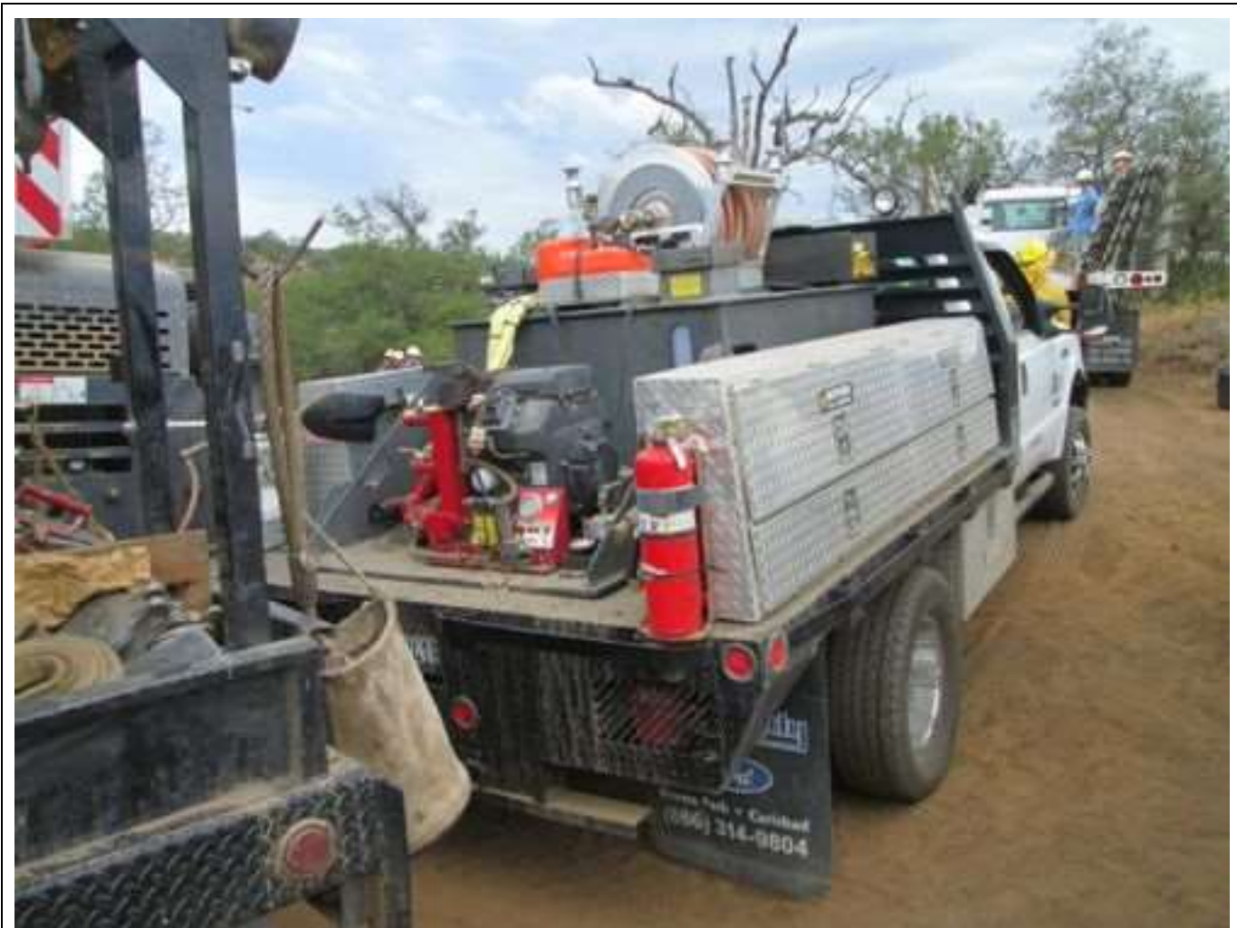
Photo 4: During micropile activities, in accordance with the Project Fire Plan and APM HAZ-2, fire suppression tools (pulaski, shovel, fire extinguisher, and 5-gallon water pump) were observed staged at work locations and carried within project vehicles. “Fire watch” individuals and response vehicles (such as a Type 6 fire engine, above) were designated and mobilized for project activities along the right-of-way.
