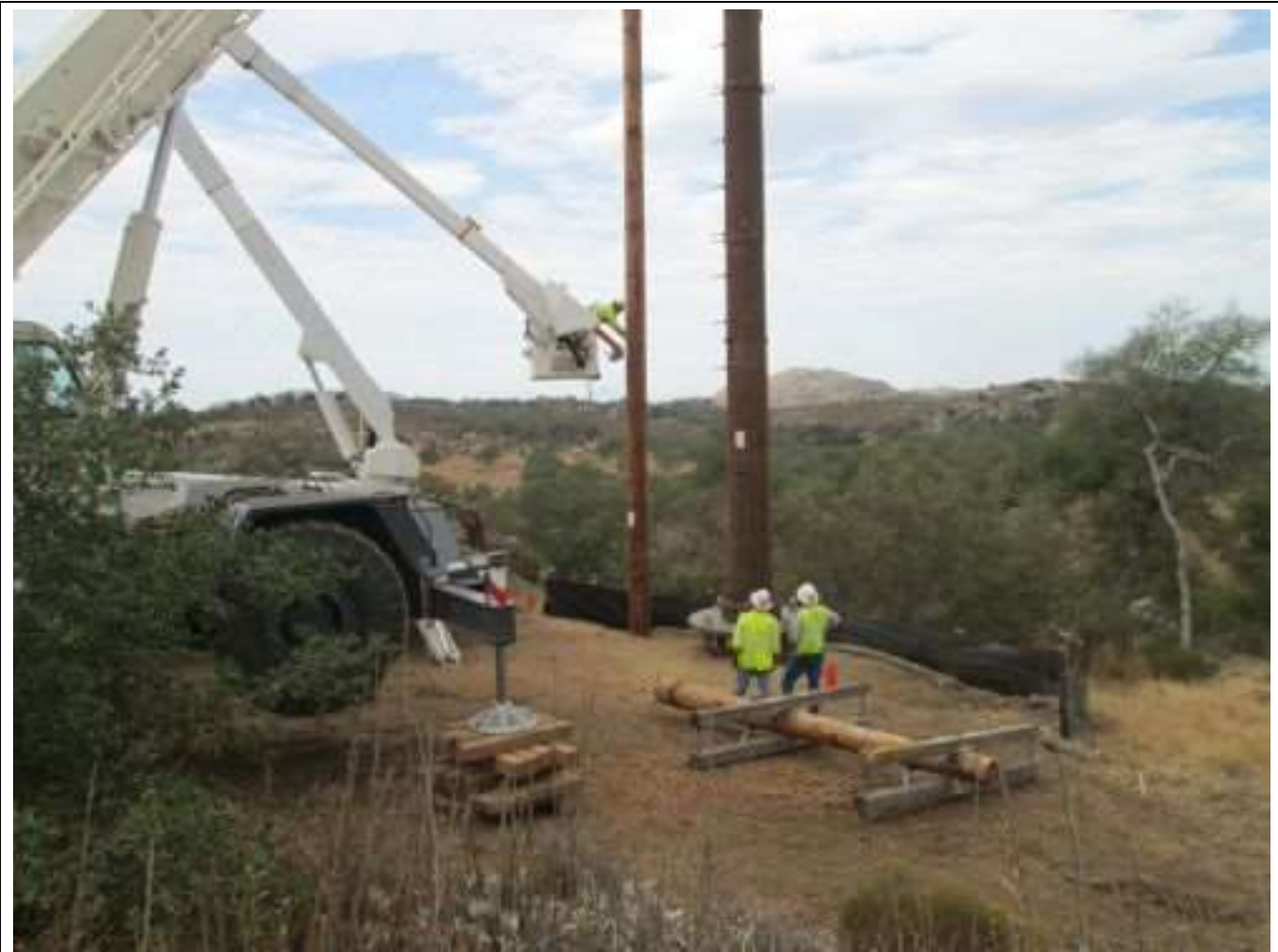
Photo 2: Crews were observed removing older wooden poles from service (left pole).
